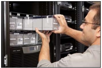
IT manager easily replacing battery module.
